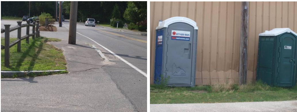
Pole obstructs sidewalk path. No HP toilets or accessible route to them.
