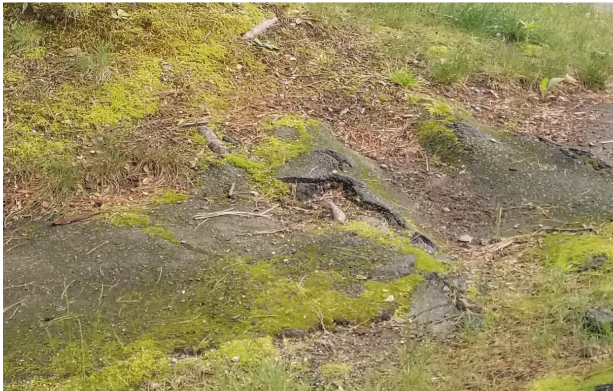
Photo 2 – Sidewalk Cracks
