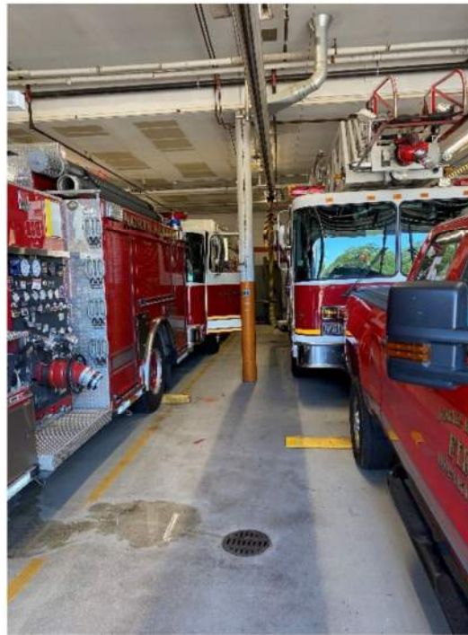
Open Doors Conflict with Structure
