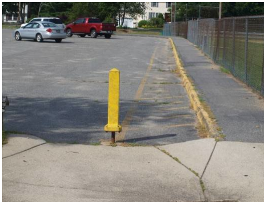
Bollard restricts access from parking area. Concession stand shelf is too high for wheelchair service.
