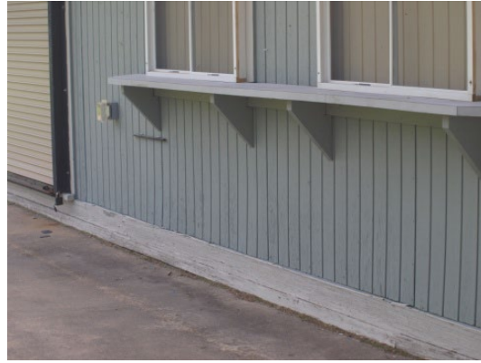
Bollard restricts access from parking area. Concession stand shelf is too high for wheelchair service.
