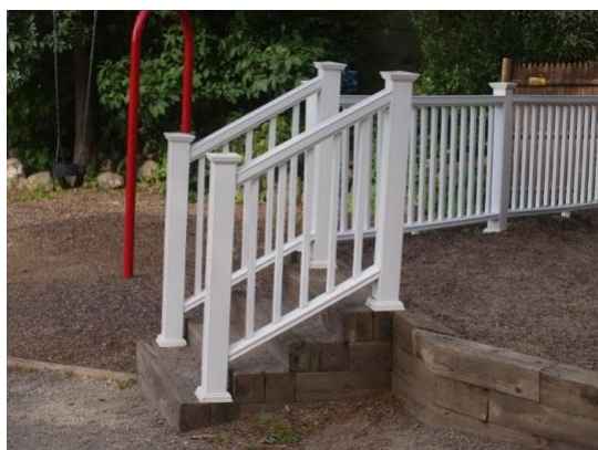
Stair railings do not meet ADA standards.
